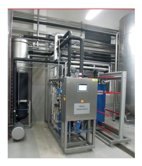
Stripping technology for deaerated water production with water sterilization
