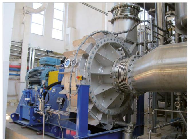
Fig. 5: Ventilator compressor in an evaporation plant.
