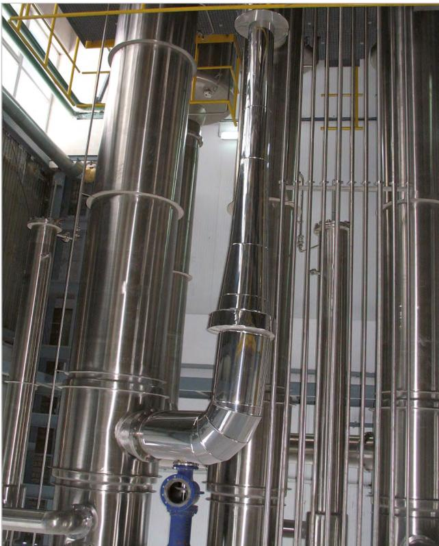
Fig. 3: Evaporation stage with TVR (thermal vapour recompression)
